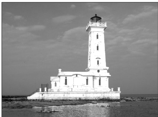
Point Abino Lighthouse, a beautiful Greek Revival tower built near Fort Erie, 1917.
